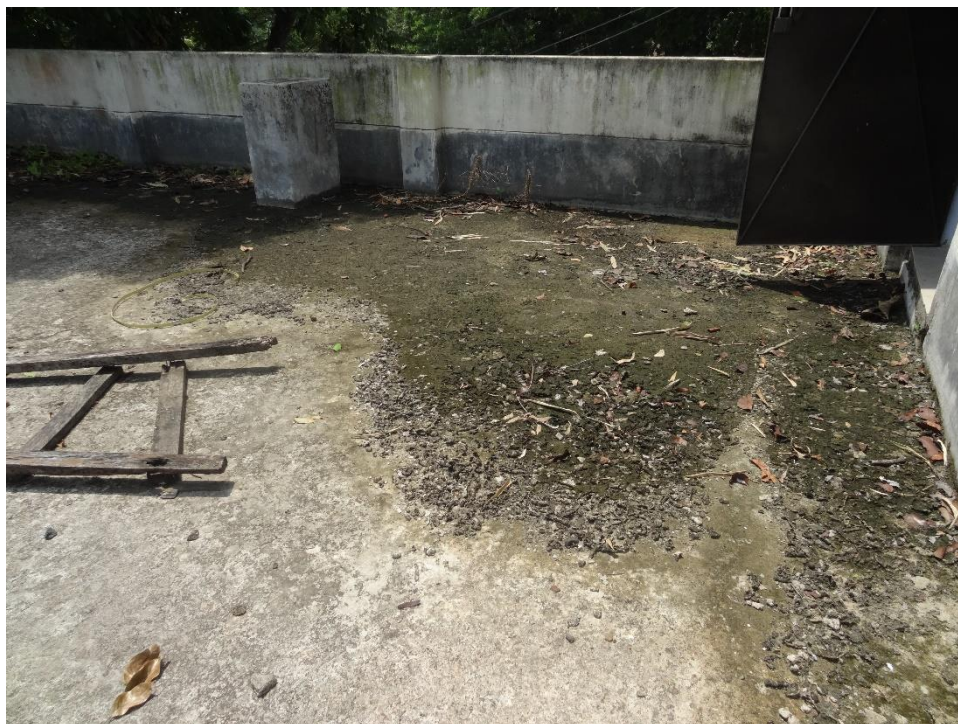
Figure 6.5: Existing Condition of Roof Slab
