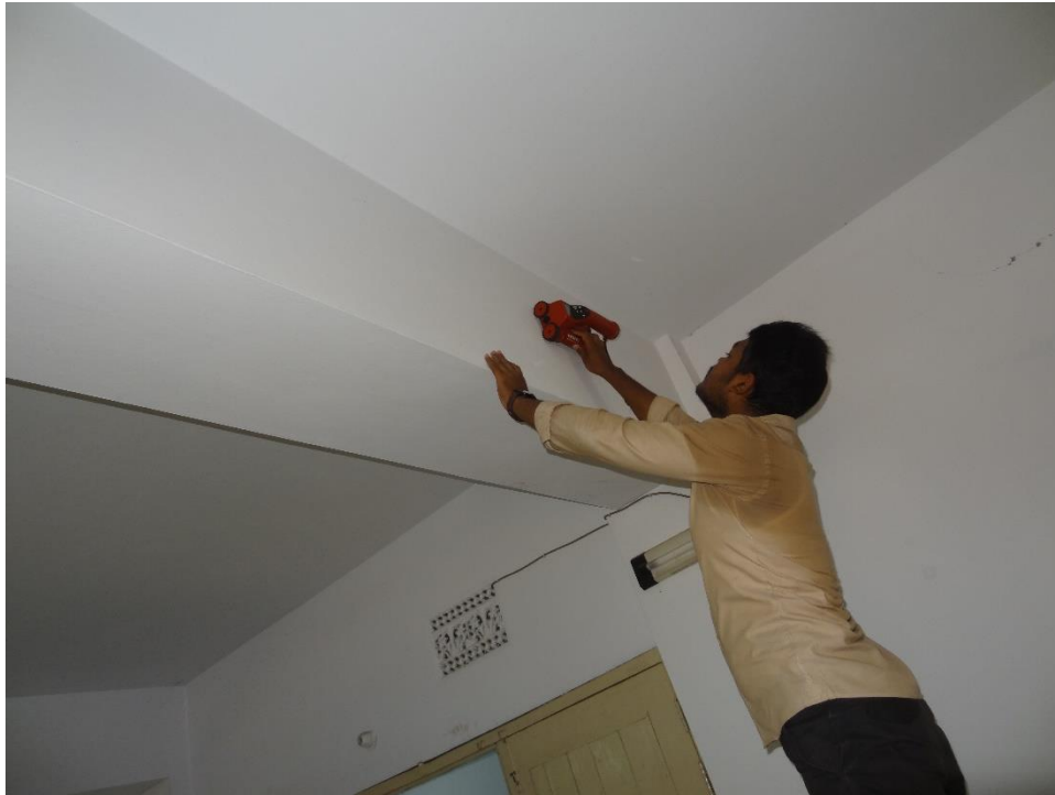
Figure 6.3: Checking of Beam Reinforcement and spacing
