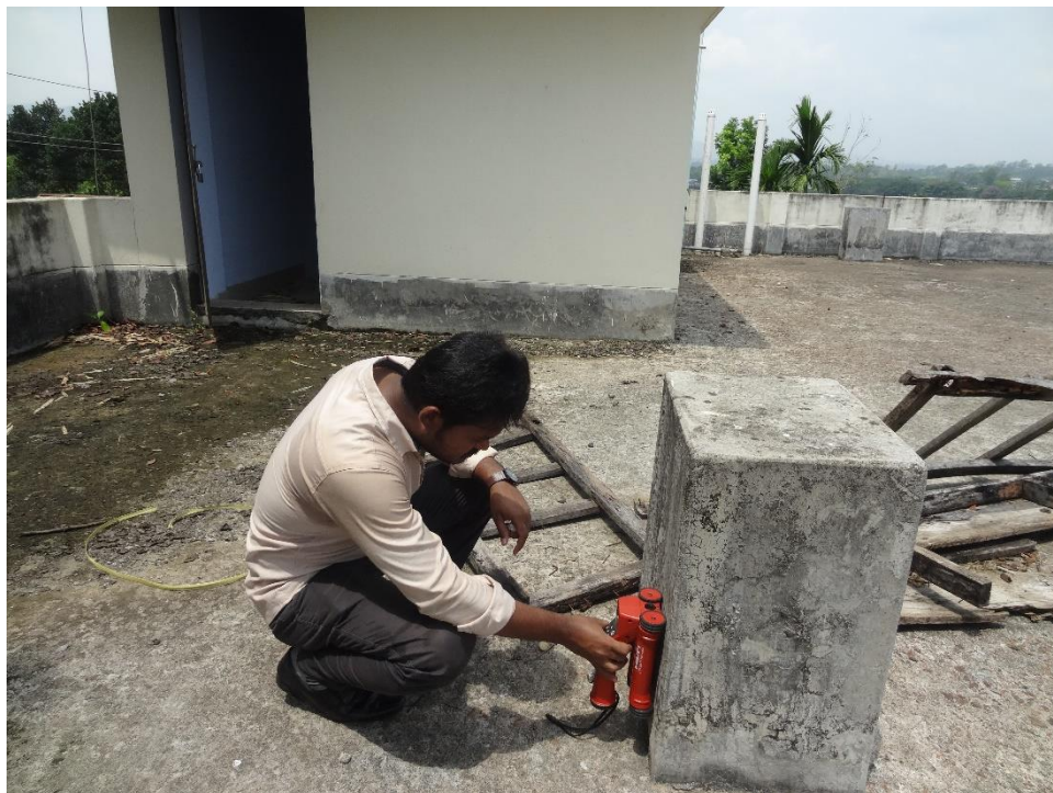
Figure 6.2: Checking the Column Reinforcement
