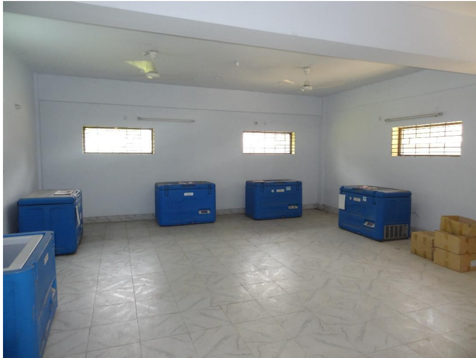
Figure 6.8: Existing condition of Cold Room at Ground floor
