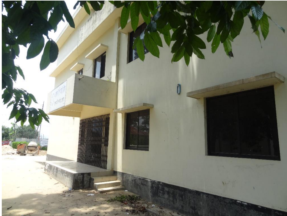
Figure 6.11: Front side Building Condition
