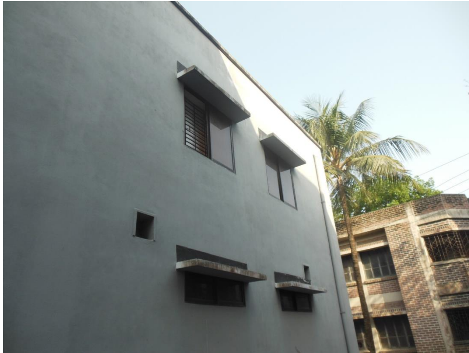
Figure 6.5: Backside condition of building
