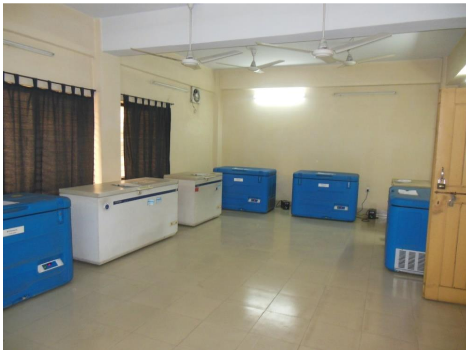
Figure 6.6: Existing Vaccine Storage Room Condition (ground floor)
