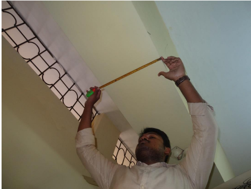
Figure 6.4: Measuring Beam Dimension
