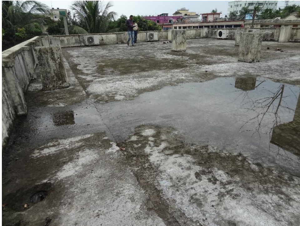
Figure 6.6: Existing Condition of Roof Slab
