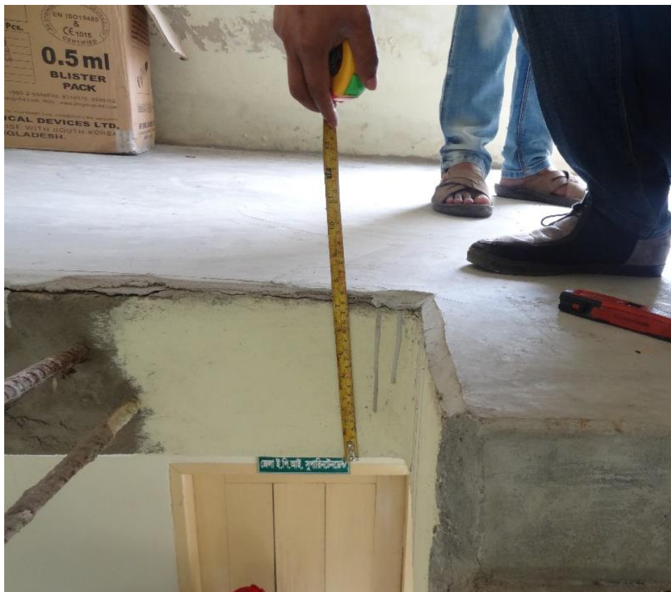
Figure 6.5: Measuring Waist Slab Thickness
