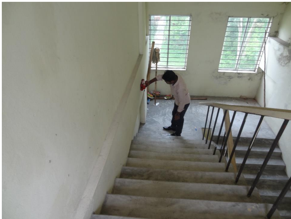
Figure 6.3: Checking of Beam Reinforcement and Stirrup Spacing
