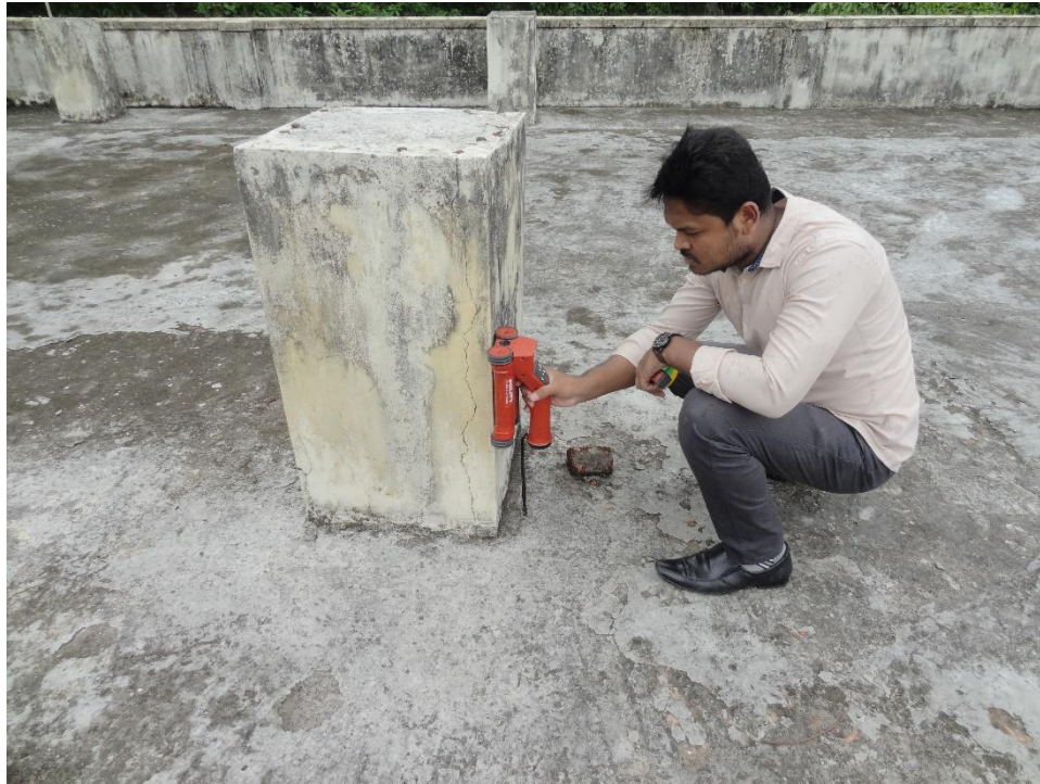
Figure 6.2: Checking of Column Reinforcement and Stirrup Spacing
