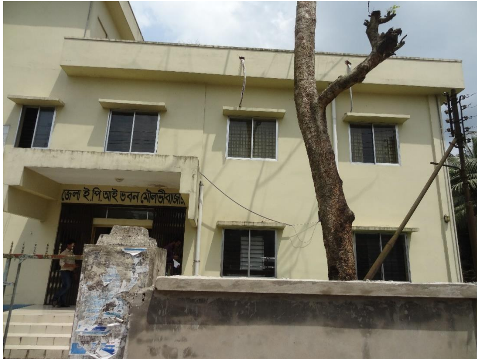
Figure 6.12: Front side Building Condition
