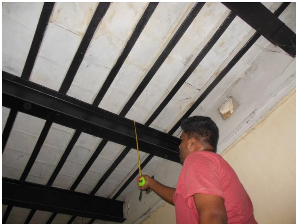
Figure 6.5: Measuring physical dimension of steel beam
