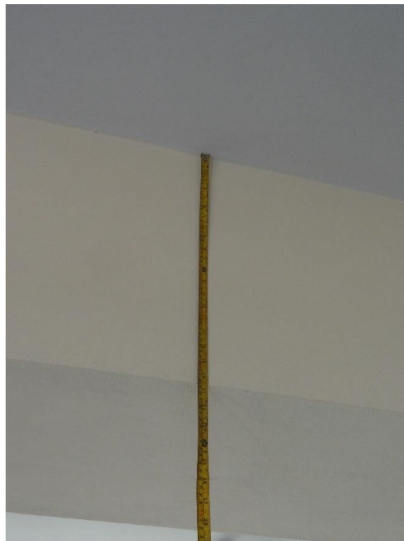
Figure 6.8: Measurement taking of beam depth (1 st floor)
