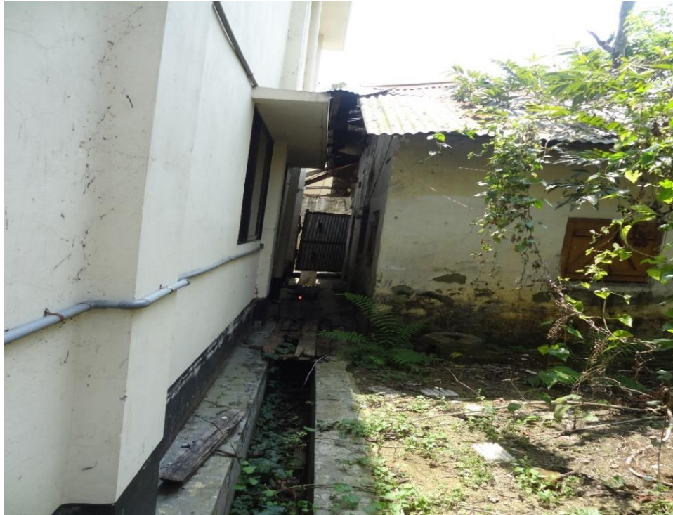
Figure 6.13: Backside Building Condition
