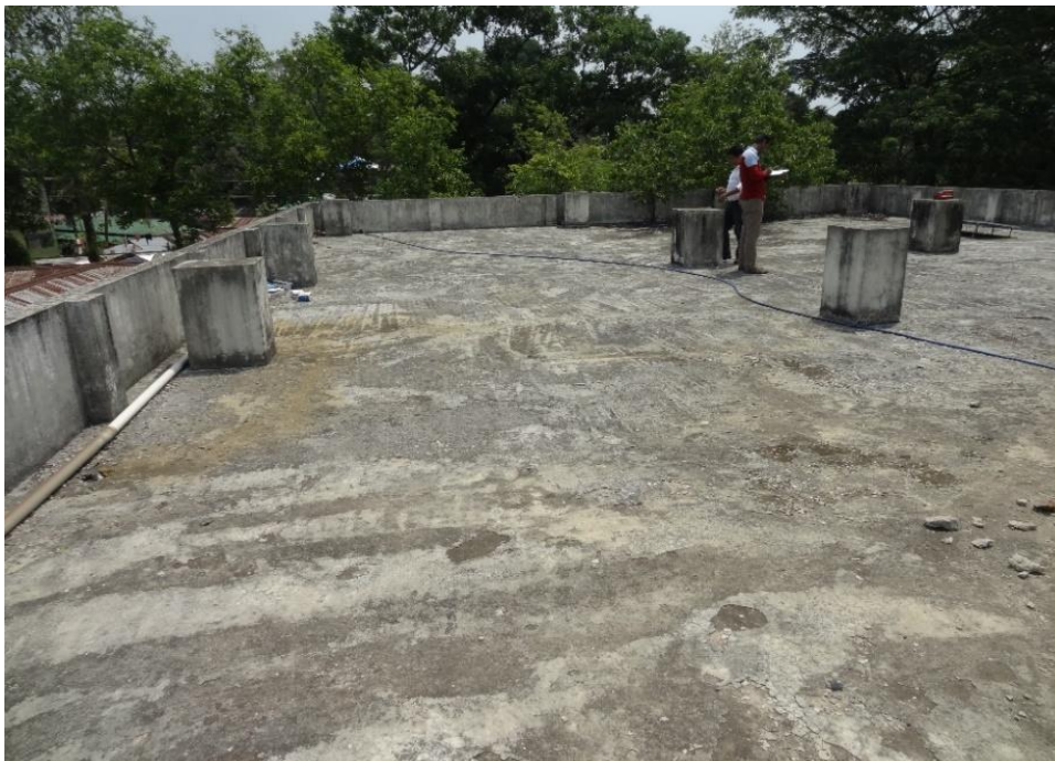
Figure 6.4: Existing Condition of Roof Slab
