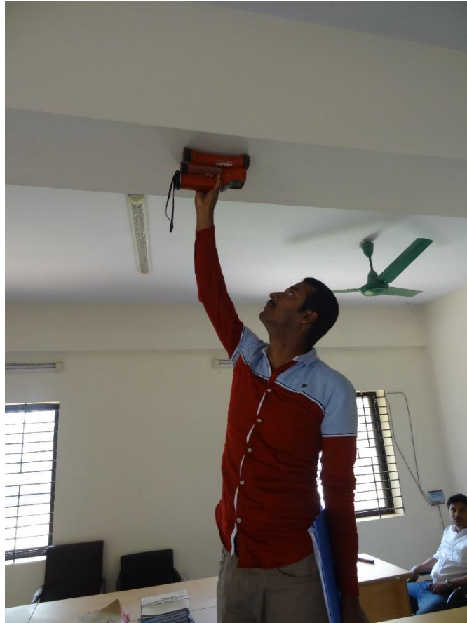
Figure 6.3: Checking Beam Reinforcement and Spacing
