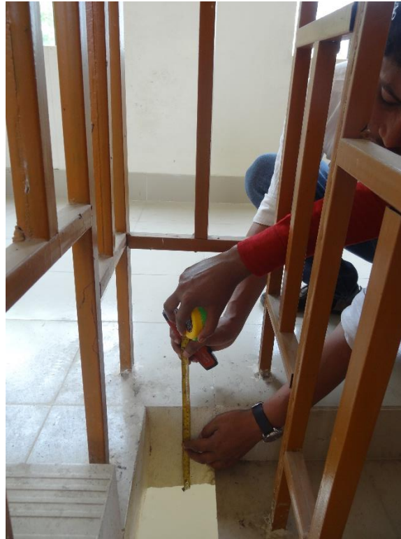
Figure 6.9: Measurement taking of waist slab thickness (1 st floor)
