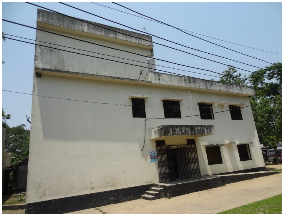
Figure 6.12: Front side Building Condition
