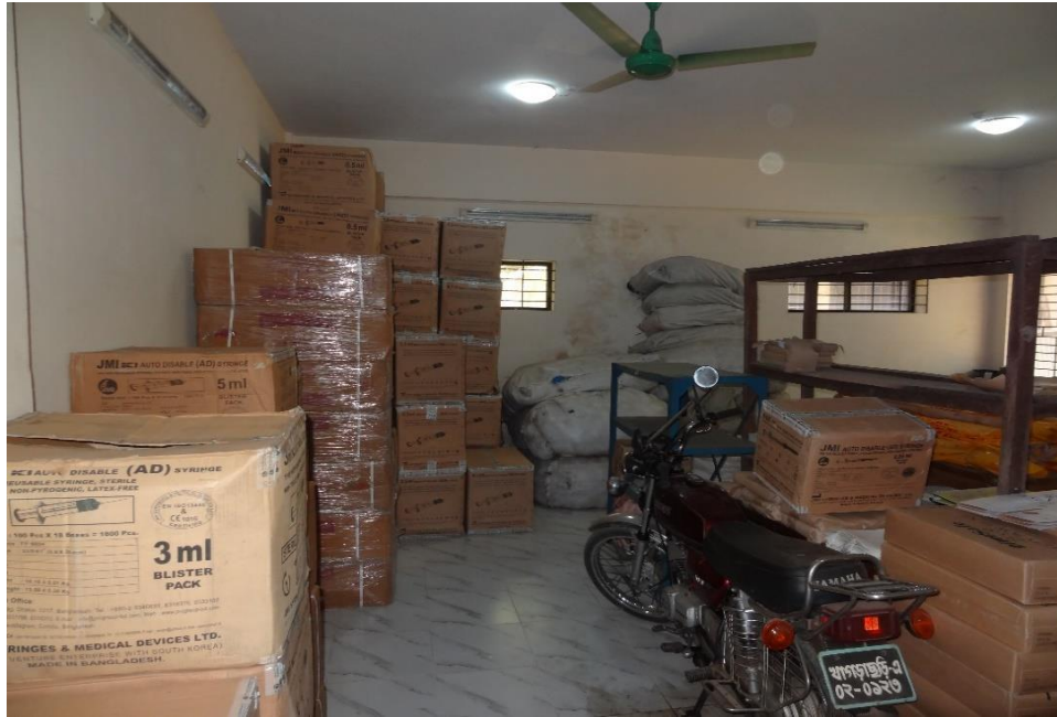
Figure 6.11: Existing Condition of Logistic Room at Ground floor
