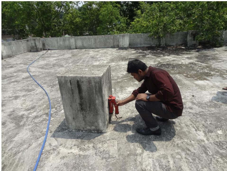
Figure 6.2: Checking Column Reinforcement and Spacing
