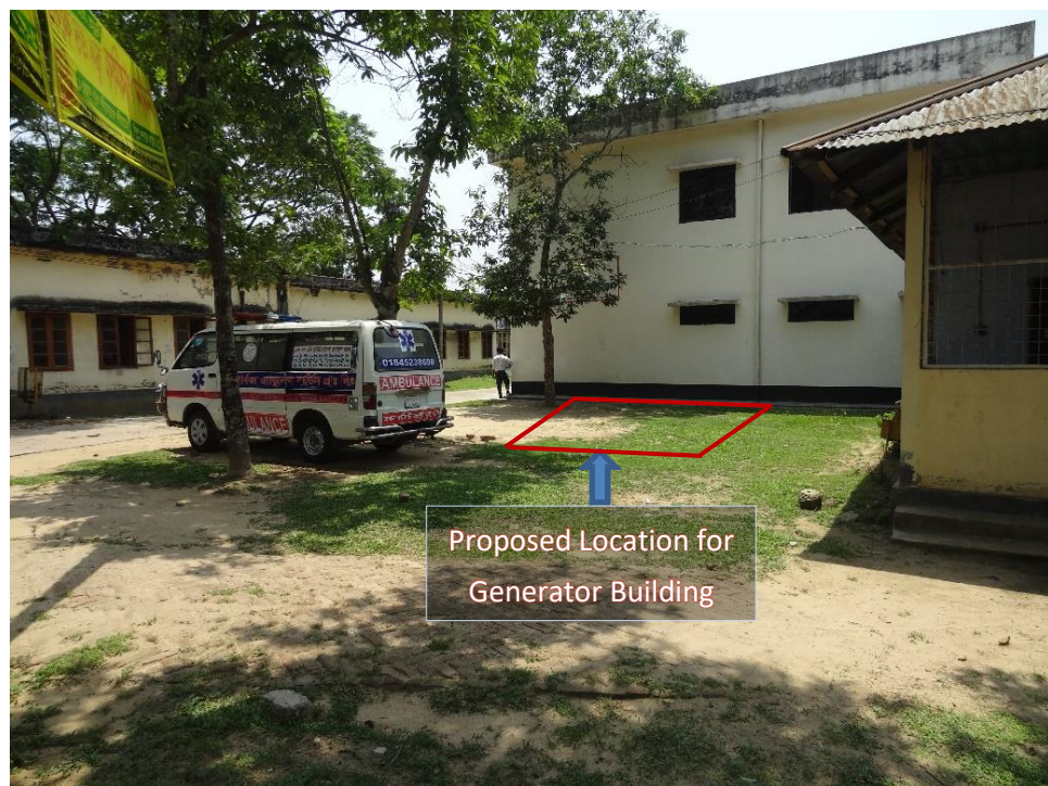
Figure 8.1: Proposed land for new generator room construction.
