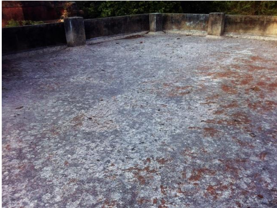
Figure 6.5: Existing roof condition
