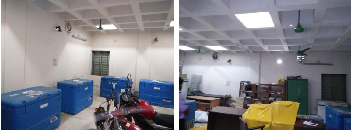
Figure 6.9: Existing vaccine storage room
